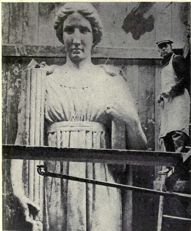
FIG. 43—FINISHING CLAY MODEL 16' HIGH FOR CONCRETE STATUE
